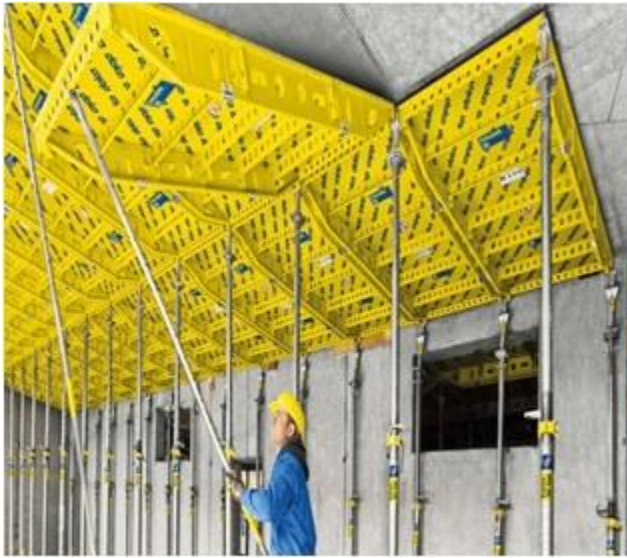
Slab Formwork Removal
