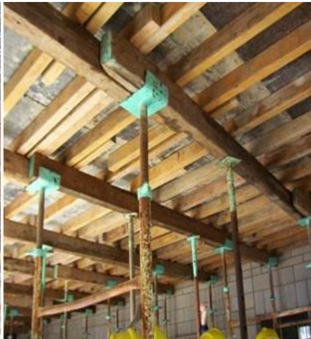
Slab Formwork made of Wood
