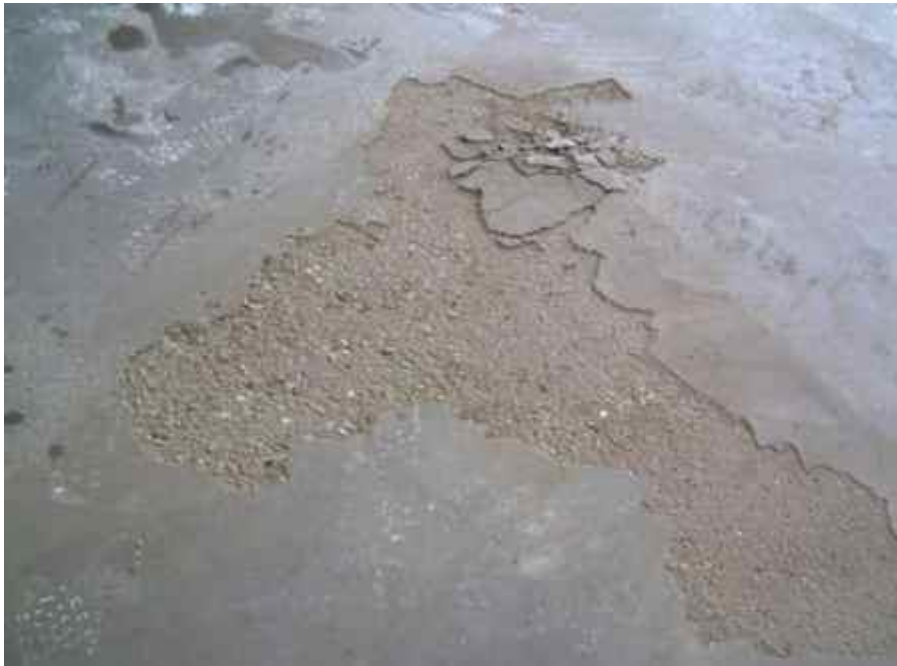
Fig 4: Delamination
