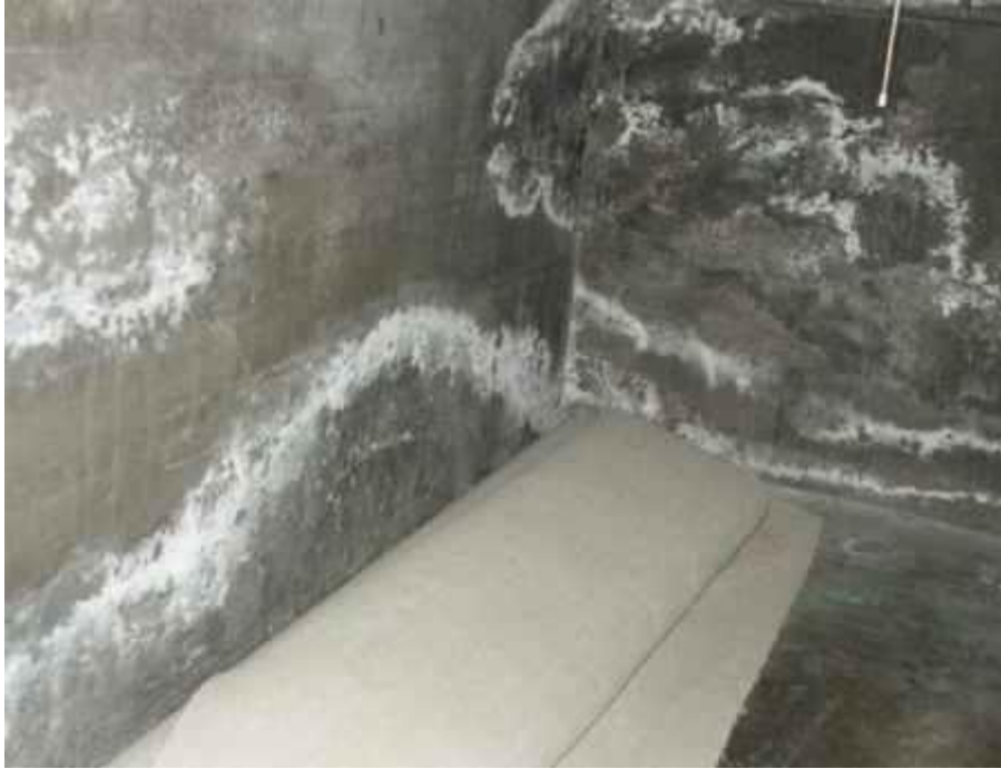
Fig 7: Efflorescence
