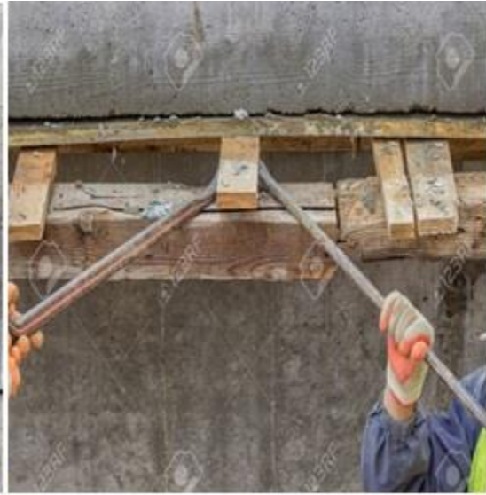
Formwork Removal with Crowbar
