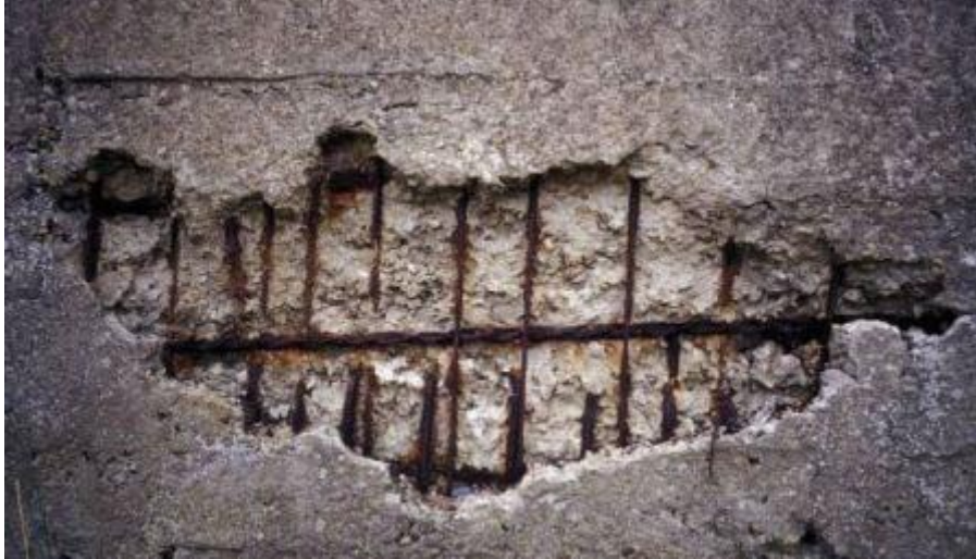
Fig 9: Spalling
