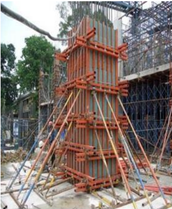
Column Formwork made of Steel
