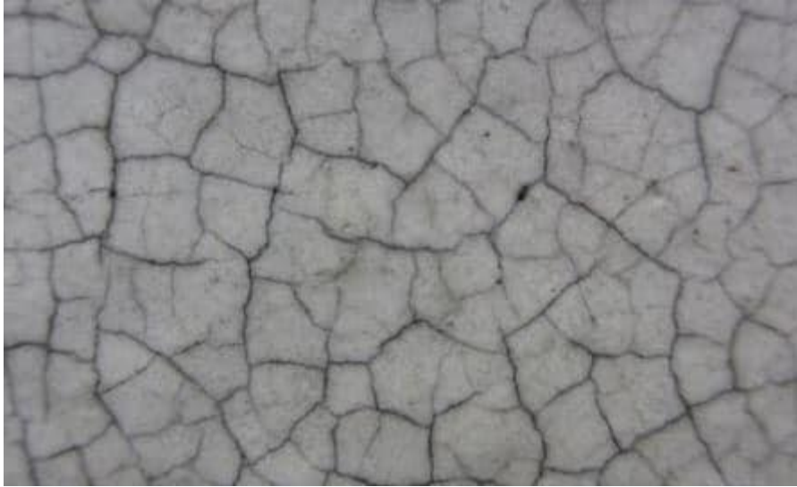
Fig 2: Crazing or Pattern Cracking
