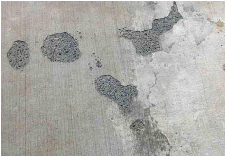
Fig 3: Concrete Blisters
