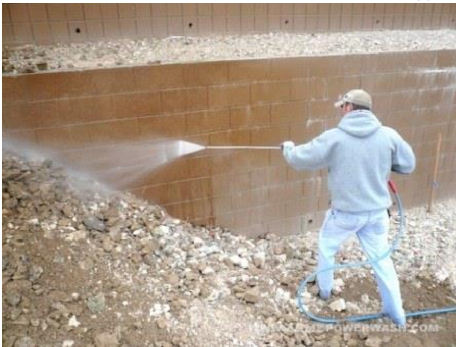
efflorescence using pressurised water.
