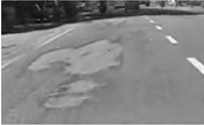
Fig.4: Semi-Dense Bituminous Concrete Highways with Shallow Potholes
